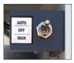
The AUTO/OFF/MAN switch should stay in the AUTO position, regardless of whether you are using main power or generator power.
